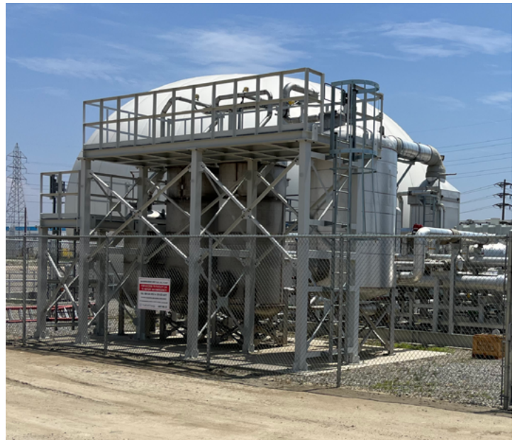
FuelCell Energy's biogas conditioning system.
